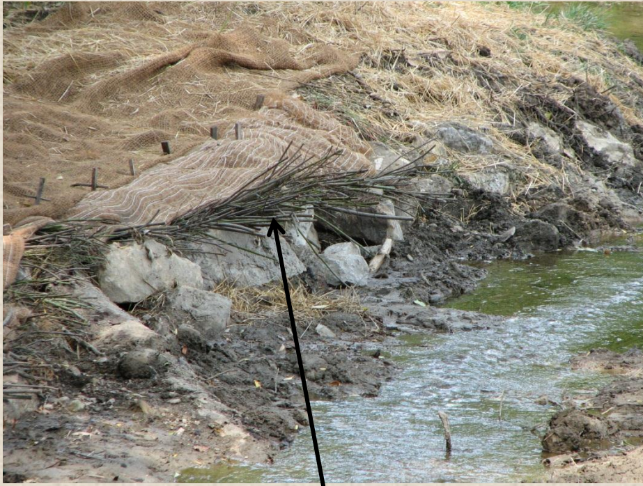
Brush Matting – placing live twigs to grow and maintain bank integrity
