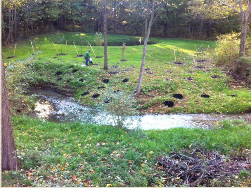
Vegetative Planting – holds bank in place
