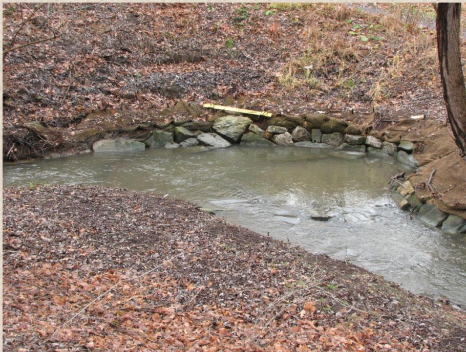
Armoring – stabilizing the streambank in a meandering form with embedded rocks
