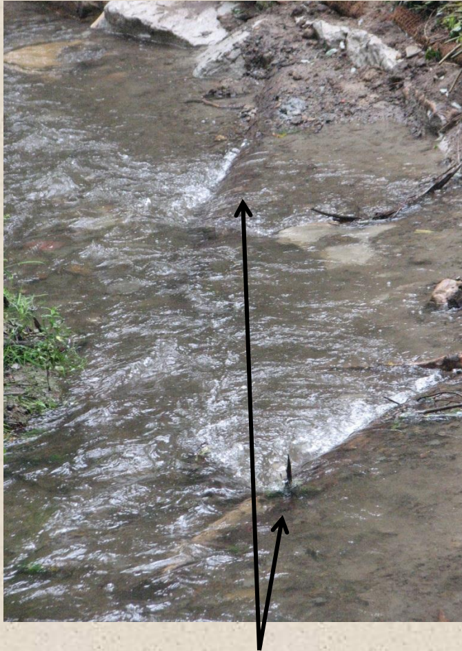
Log Vanes – deflects water from eroding the banks
