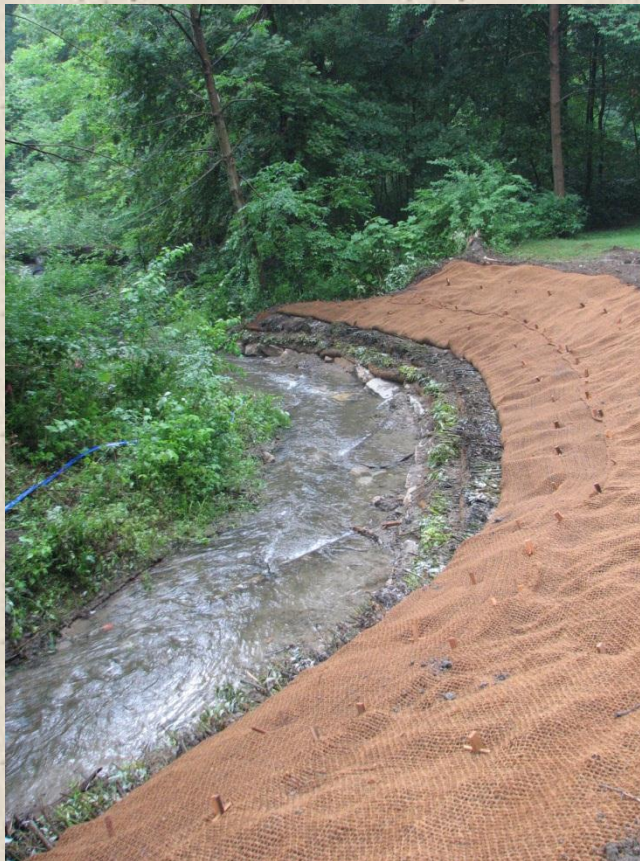
Bank Grading – eases slope, slows erosion
